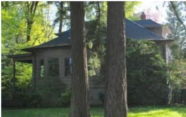
3533 SW Blackstone Lane before reconstruction
